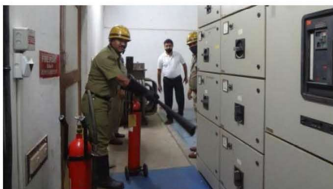
Fire mock drill at magnet power supply unit of Indus-1.
