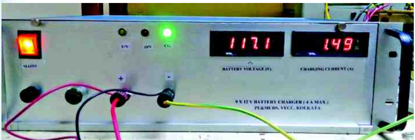
Figure 1 : Front panel of the battery charger during testing
