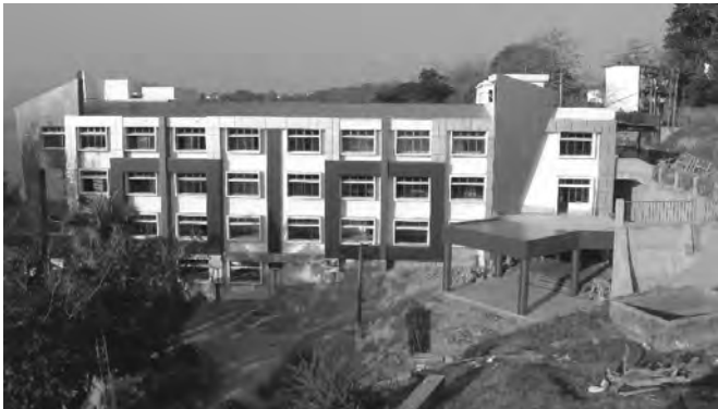
ANCOST Laboratory Facility
