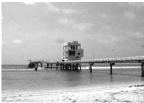
Desalination plant at Agatti
