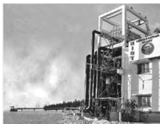
Desalination plant (LTTD) at Kavarrati Island
